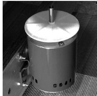
*Fan motor securely mounted to channel rail.*
